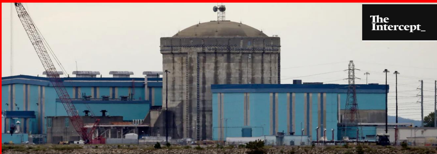
Unit one of the V.C. Summer Nuclear Station near Jenkinsville, S.C., photographed on Sept. 21, 2016. Photo: Chuck Burton/AP
