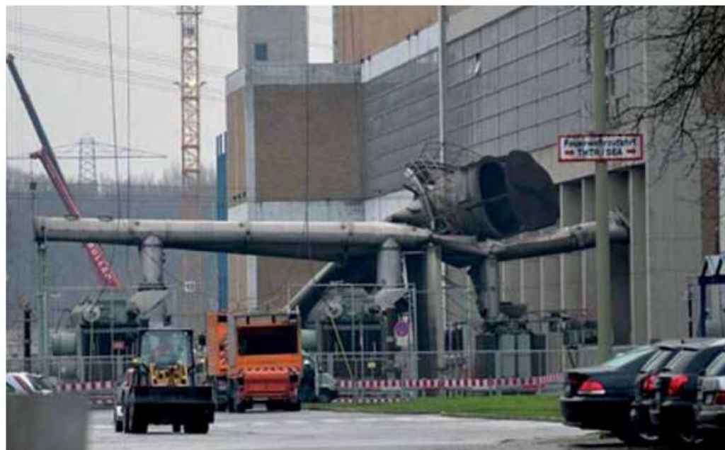
Photo 7.16 The Hamm pyrolysis stack corroded and collapsed in 2009. It was never rebuilt. Photo: Reiner Mors, tz.de, Source (dpa, 2009).
