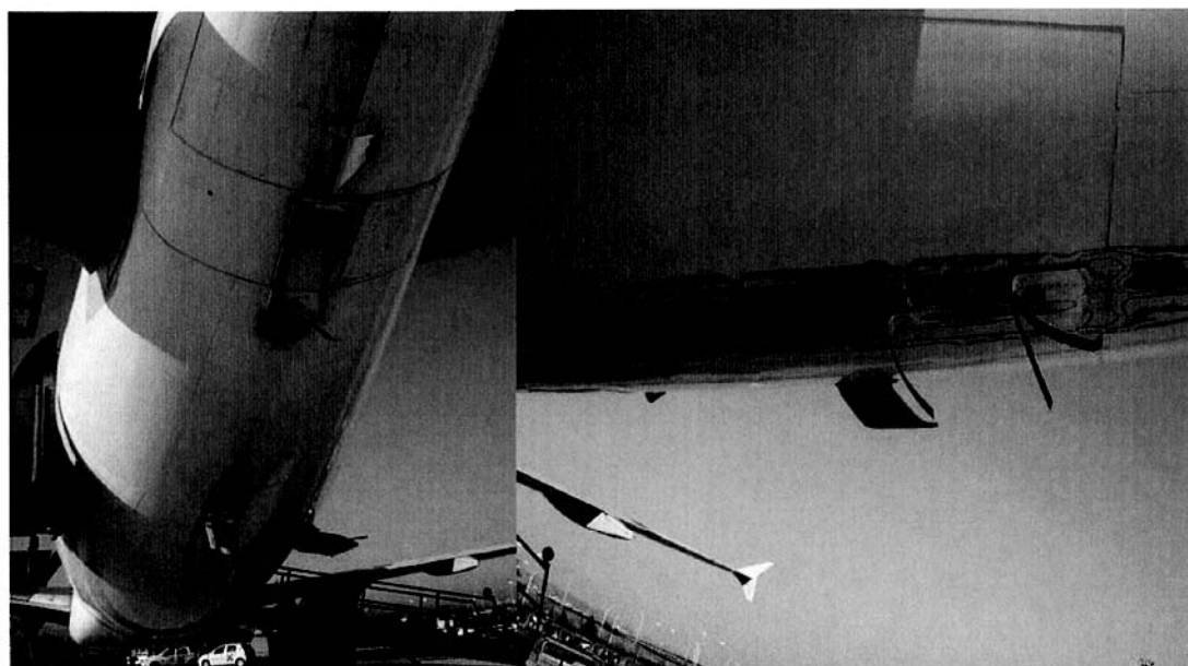
LZ-BHC: extensive structural damages to the lower part of the tail fuselage.
